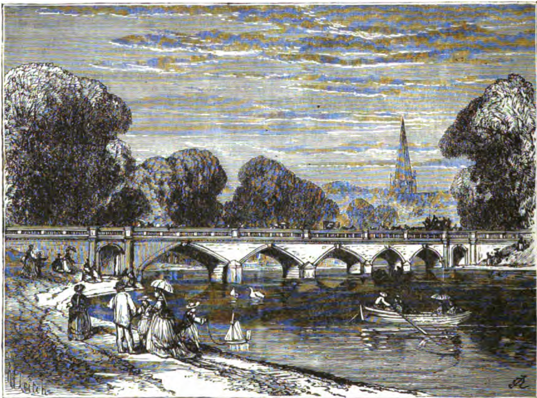
THE SERPENTINE BRIDGE.
